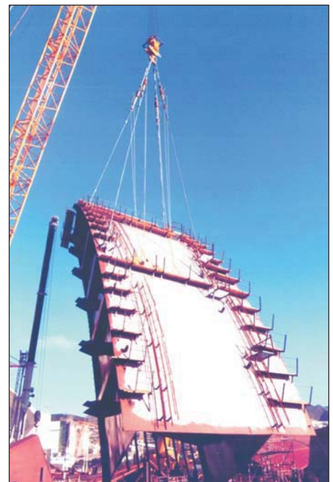
▼ Roof lifting using a 4-point Enerpac hydraulic SyncHoist System.
